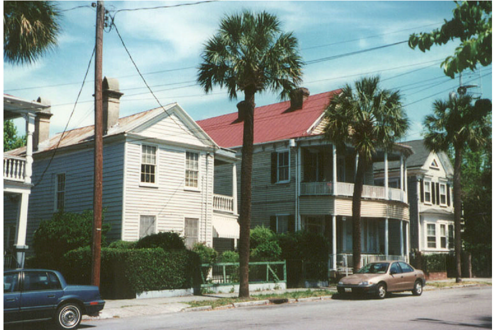
Historic Wood Frame Building in Charleston
