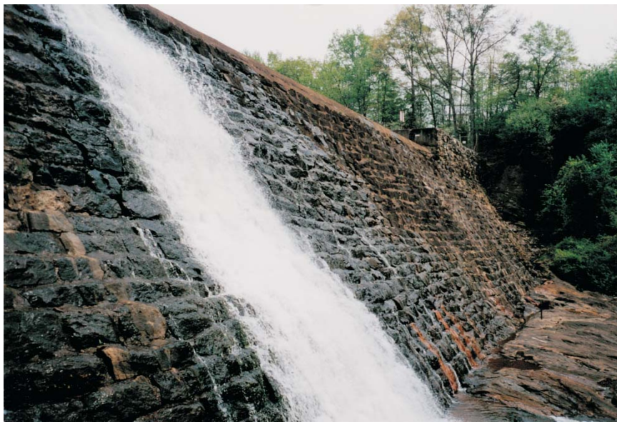
Lake Apalache Dam, Spartanburg County [Masonry Gravity]
