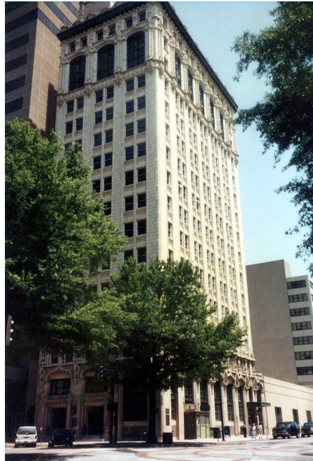
Frame with URM infill
